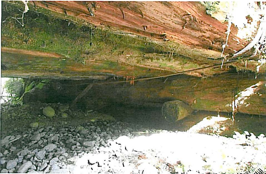
CK-2264 Left Abutment
