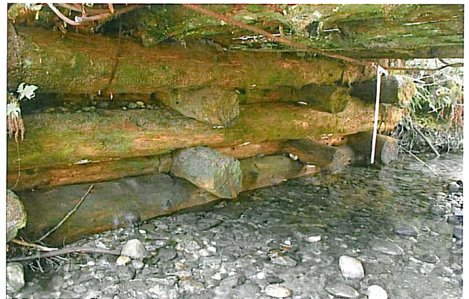
CK-2264 Right Abutment
